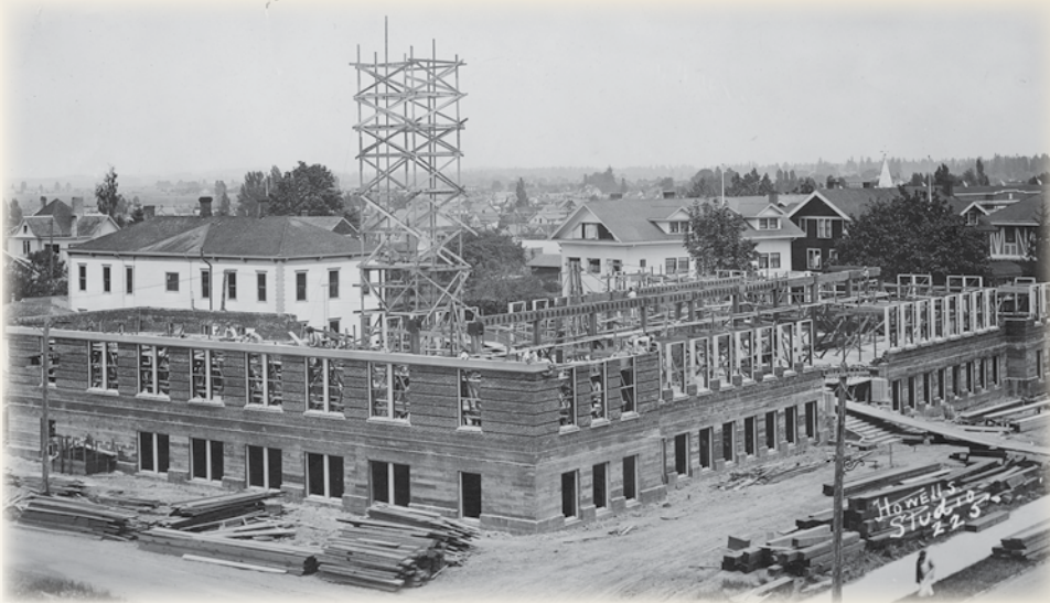
Commerce Hall under construction, with the two white sections of Alpha Hall shown to the left. Shepard Hall is shown east of Commerce Hall and Sigma Phi Epsilon and Sigma Chi houses are between Shepard Hall and Commerce Hall. The spire of the church on Monroe Street is shown in the background of the photo.
